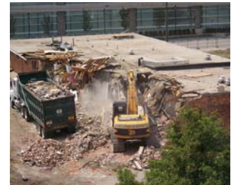
Demolition of building that housed HIA programs for 25+ years.
